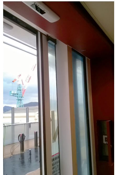
The built-in modules for door detectors feature protection against water jets and are integrated discreetly.
